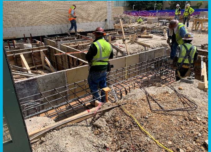
Grade Beams Installed at Kitchen Addition at Alumni Hall
