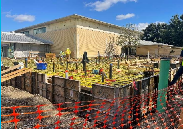
Kitchen Addition Foundation Ready for Pour at Alumni Hall
